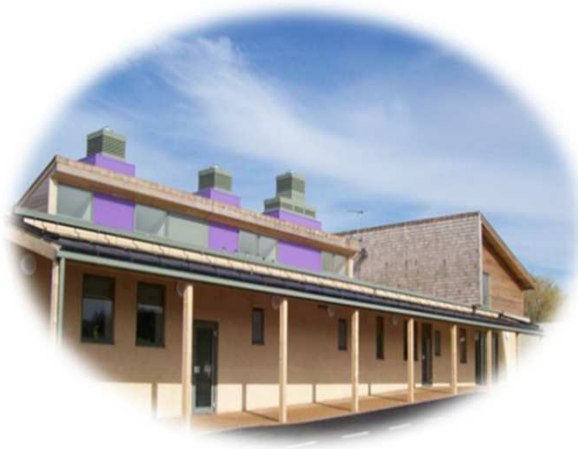
Windchimes – Herne Bay 6 Bedded Unit Jointly funded by KCC and Health Authority
